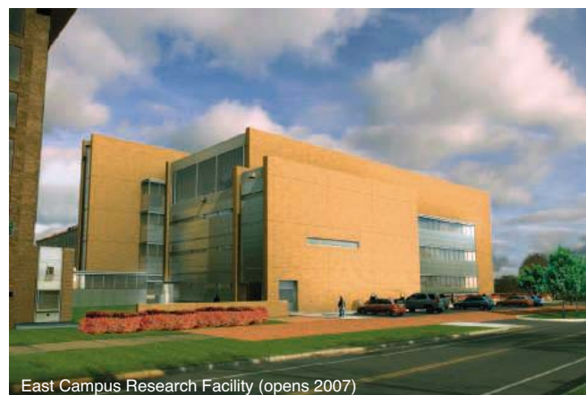
East Campus Research Facility (opens 2007)
